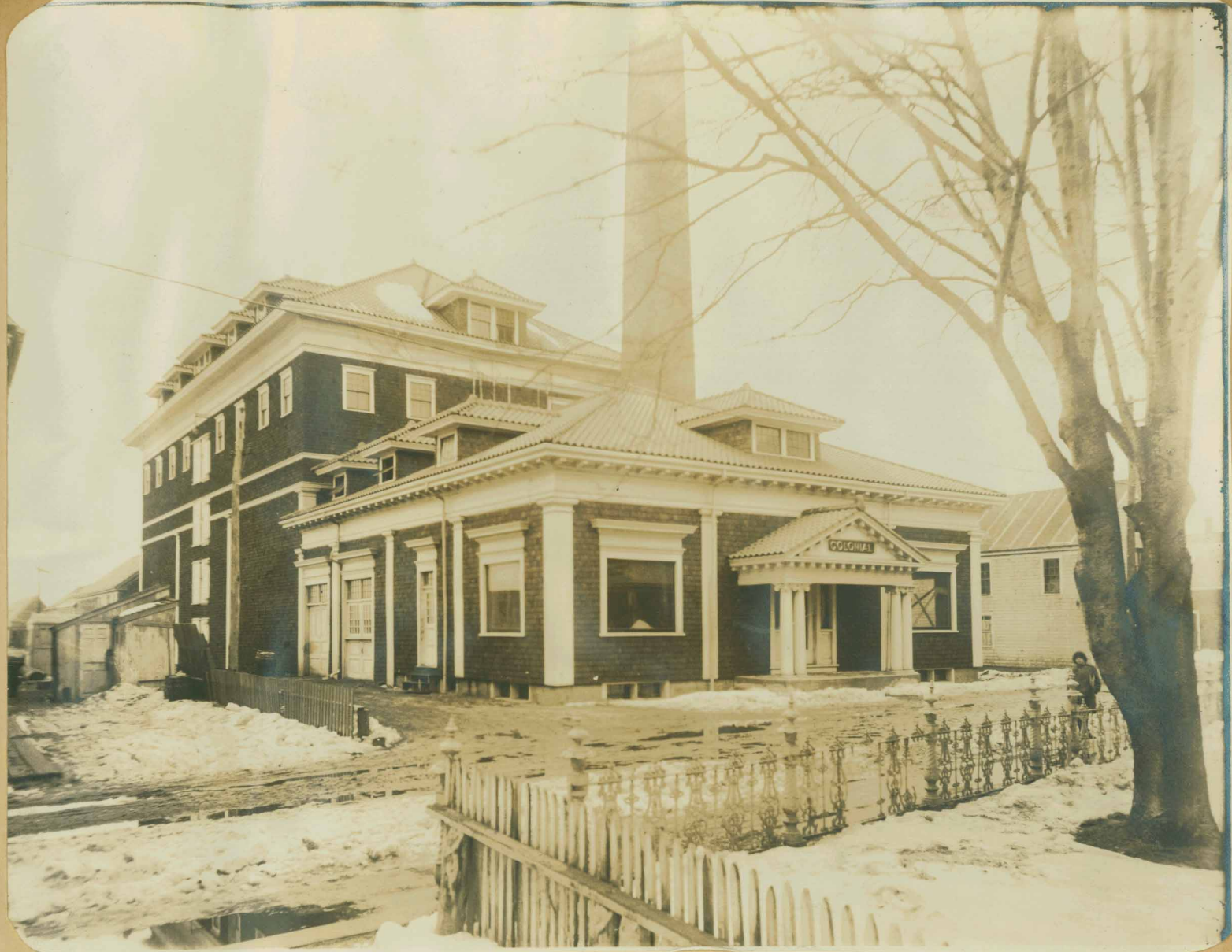
The Colonial Cold Storage, opposite the Ben Lancy House - About 1900
