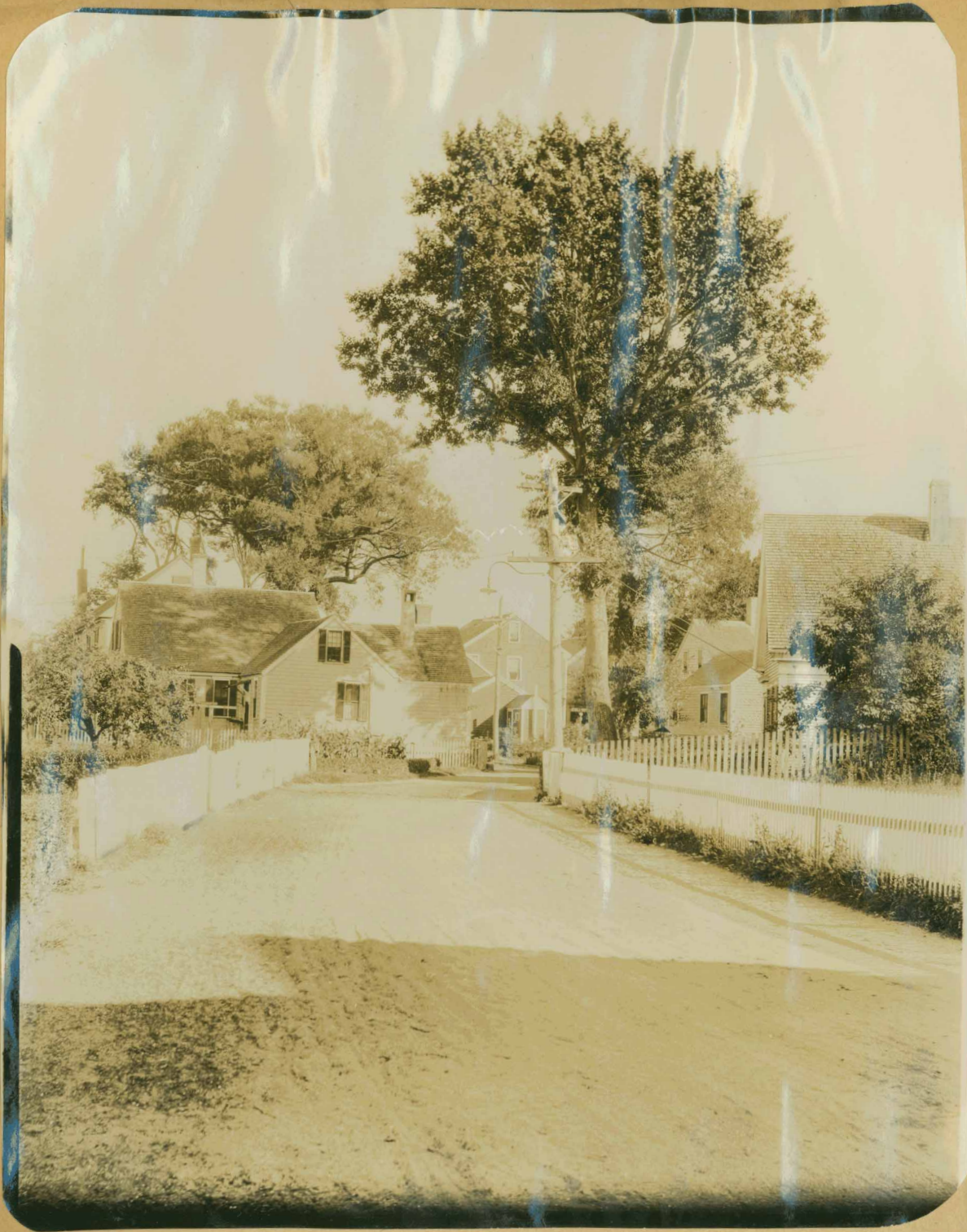
Looking up Atlantic Avenue from Bradford Street - 1915
