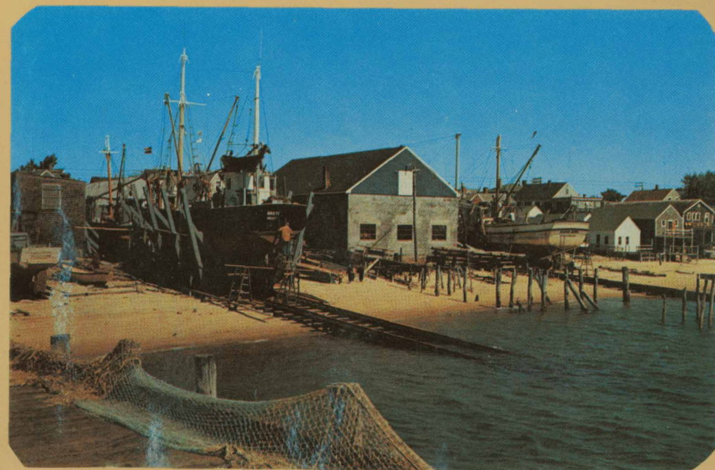
Flaves Marine Railway from the Cape Cod Cold Storage Wharf - 1957
