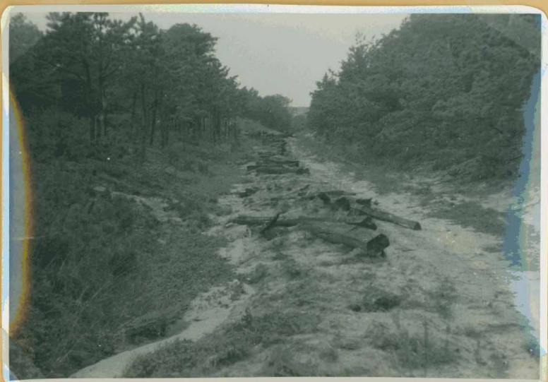
Taking up the Ties - October 1961 -
