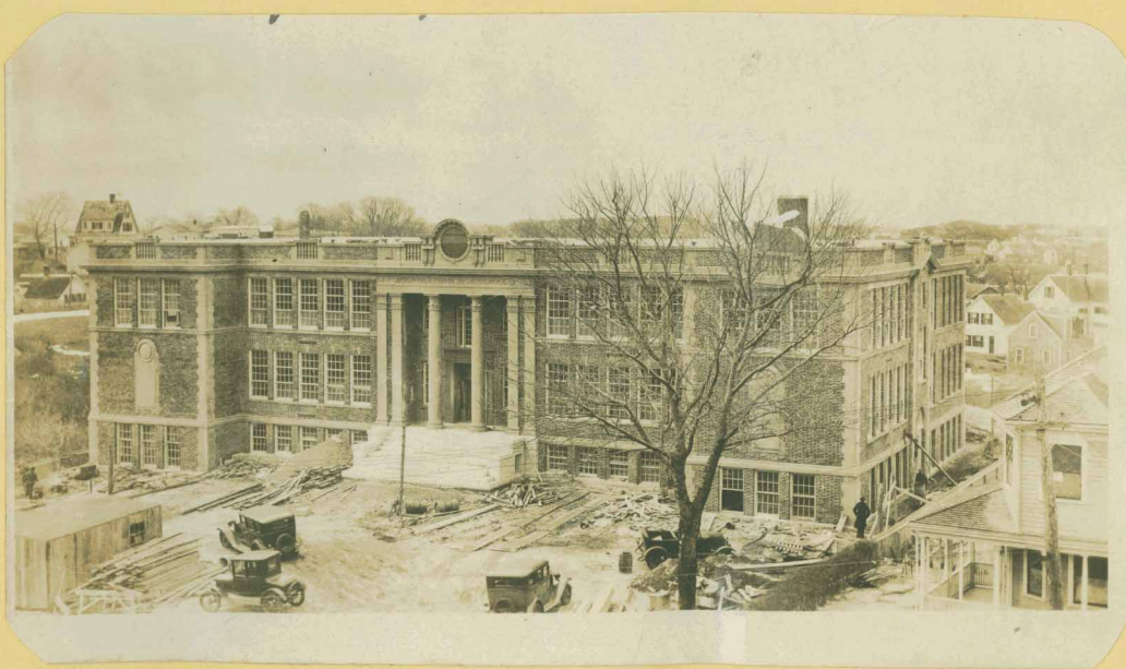
New High School going up ----- 1931
