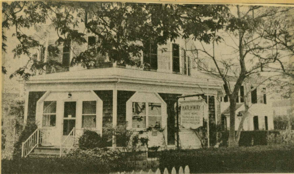
The Hatchway House, which has been forced to close by repeated demands from the state's Department of Public Safety. The house, which was built in 1834 by a whaling captain, is up for sale.
