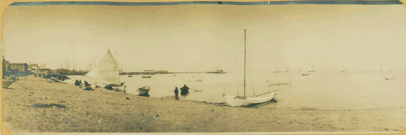
Cupola at left is the First Schoolhouse on Long Point, then was Duncan Matheson's clothing store, now Arnold's radio and appliances.
